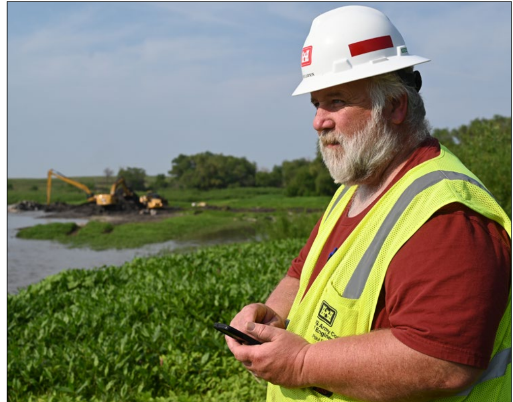
Roy Lawson, construction representative, oversees the removal of Drayton Dam, near Drayton, North Dakota, June 27. USACE St. Paul District photo by Patrick Moes
